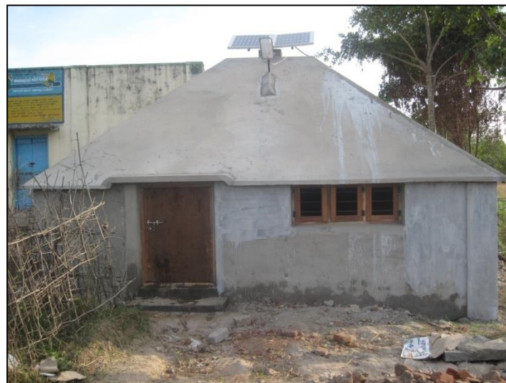
Figure 2: SPR test house
