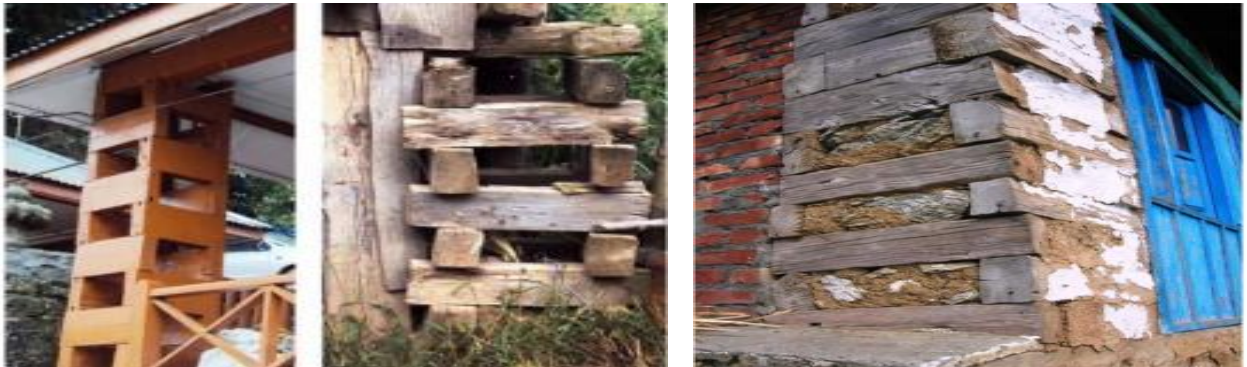
Figure 2: Frames (Thola) for Thathara construction
