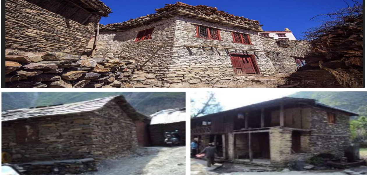
Figure 4: Dry stone constructions in Nepal and Lahoul Spiti
