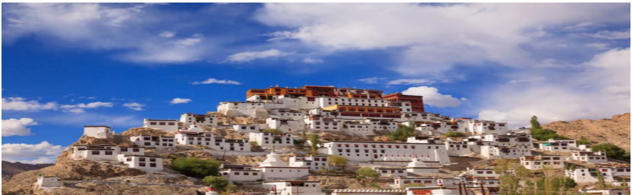
Figure 3: Mud Wall Construction of Monasteries in Ladakh
