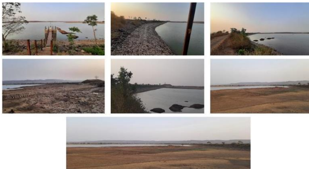
Figure 2: Some photographs of Piplod Dam, Pansemal
