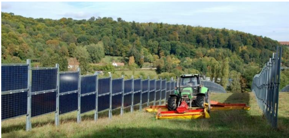
Fig. 4: Vertical Bifacial Agrivoltaic (Gupta, 2024)
